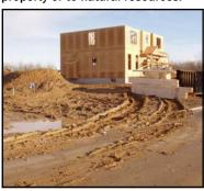
Rain could easily wash this loose soil into the storm sewer and into a nearby stream, causing a water quality standards violation that could cost the site operator up to \$37,500 each day it occurs.
